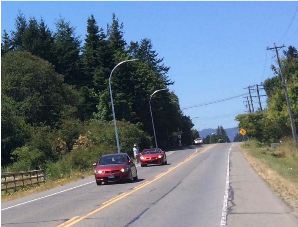
Overhead lighting and paved, wide road shoulders for improved walking and cycling safety on busy Mt. Newton X Road.
